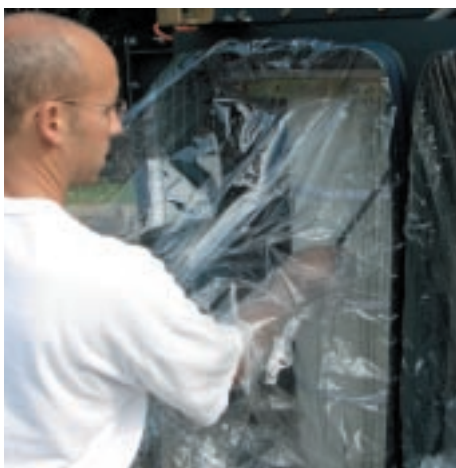
Hazardous compounds contained with BIBO filter change. Filters are sealed via cam-lock action, making it easy to work through the bag.
