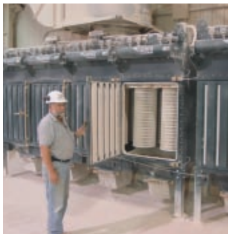
Louvered door inlet for cross-flow applications
